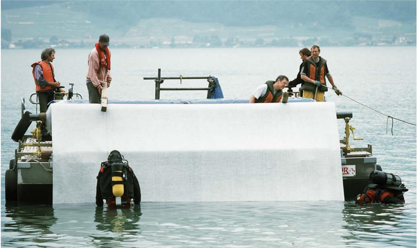
Fig. 4 Spreading of heavy geotextile mats with a sand inlay of 5 m width and 30 m length, which are normally used in road construction. The special ship of the Archaeological Service of the Canton of Bern in an operation on Lake Biel. © Archaeological Service of the Canton of Bern, diving team.
