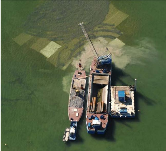
Fig. 1 Covering the archaeological site of Rapperswil-Jona, Technikum, in the shallow water zone of Lake Zurich, Switzerland, with geotextile and gravel. Use of a gravel barge and a crane with jib. © Archaeological Service of the Canton of St. Gallen, Simon Vogt, 2011.
